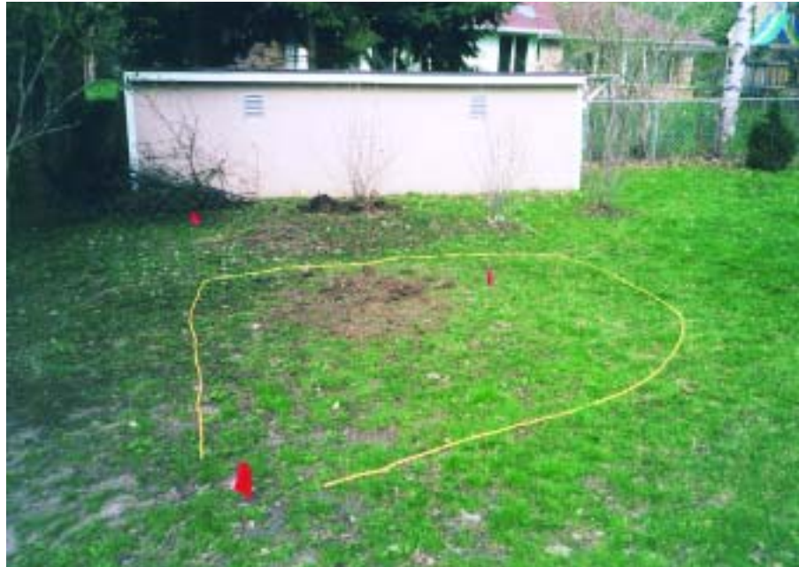
The perimeter of a rain garden is defined with string before digging.
