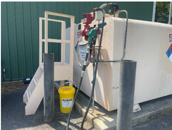
Figure 5. Spill kit at Township vehicle fueling station
