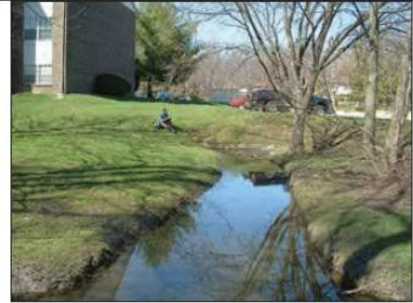
Fully submerged: Can't see outfall
